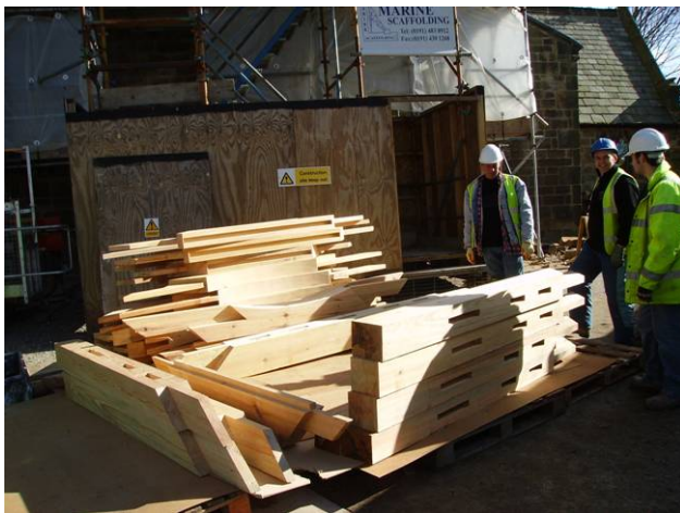
Figure 8 & 9 The pitch pine trusses were delivered as the worst flat-pack nightmare. The spire was constructed without difficulty on site using Douglas Fir, although this was imported rather Scottish..
