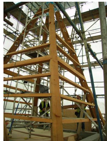
Figure 8 & 9 The pitch pine trusses were delivered as the worst flat-pack nightmare. The spire was constructed without difficulty on site using Douglas Fir, although this was imported rather Scottish..
