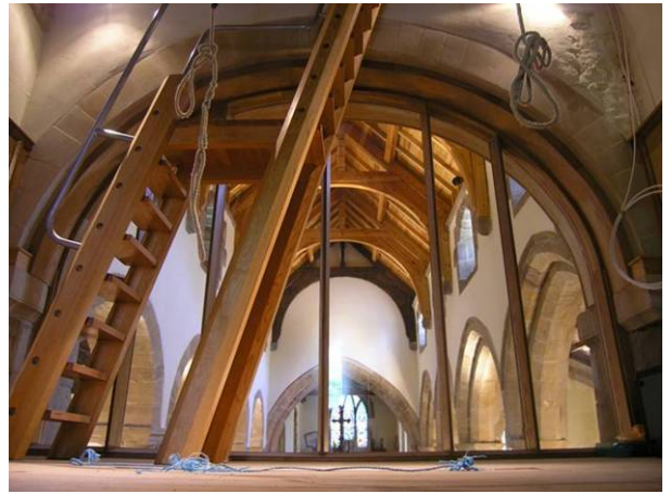
Figures 6 & 7 New trusses constructed in Caribbean pitch pine as no British dry beech or ash was available. Note connections in timber.
