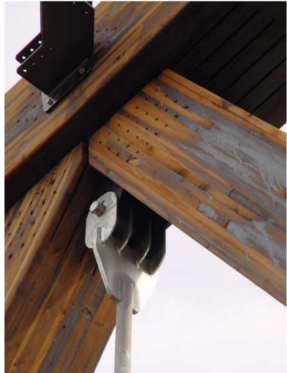
**Figure 7: Truss connection of creosoted glulam in the Flisa roadbridge, Norway**
