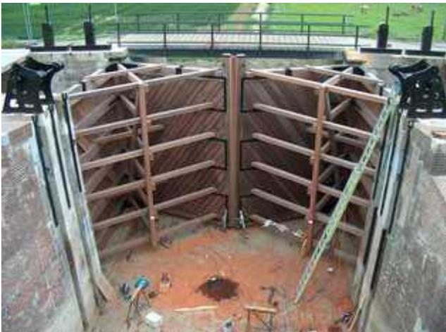
**Figure 15: Wing gates in dry condition**
