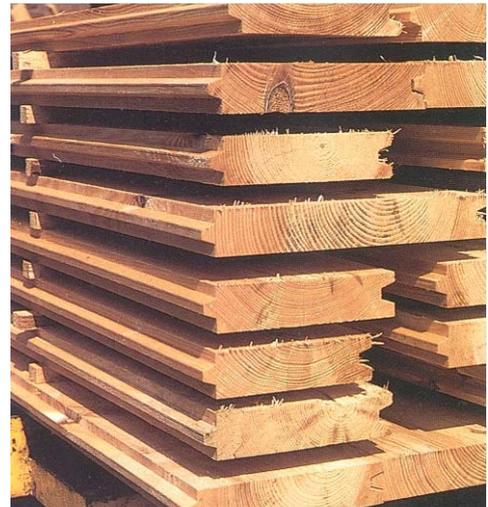
***Figure 3: Tongue and groove profile of sheet pile wall boards***
