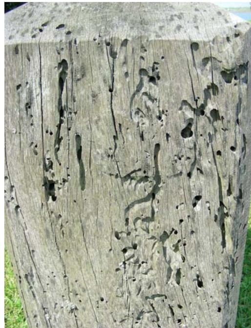
**Figure 5: Decay pattern of shipworm**
