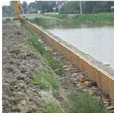
**Figure 9: Tie rods for anchor plates**
