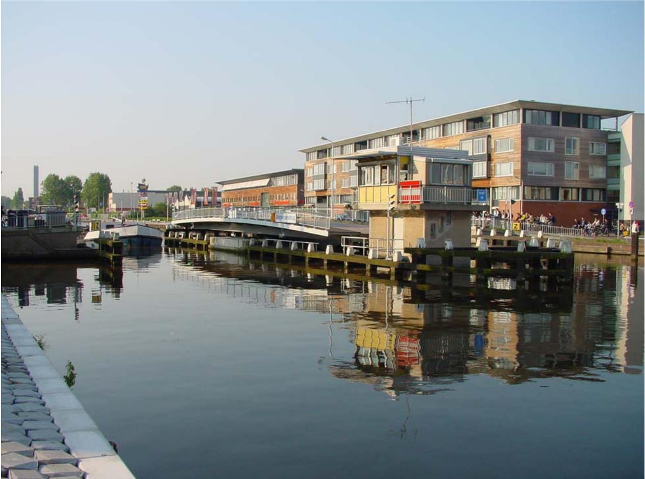
*Figure 20: Swing bridge in Delft, the Netherland, protected by timber fender structures*
