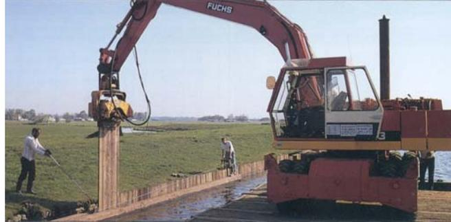
**Figure 8: Placement of a sheet pile wall by means of vibration.**
