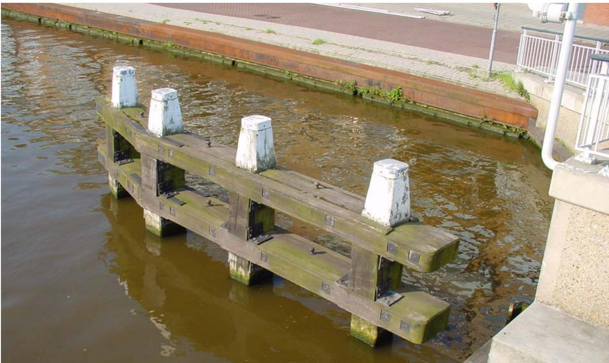
*Figure 21: Fendering structure to protect the bridgehead*
