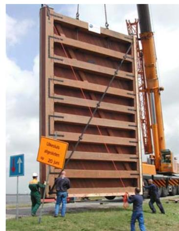
*Figure 1: Manufacturing and stepping in of hardwood lock gate*
